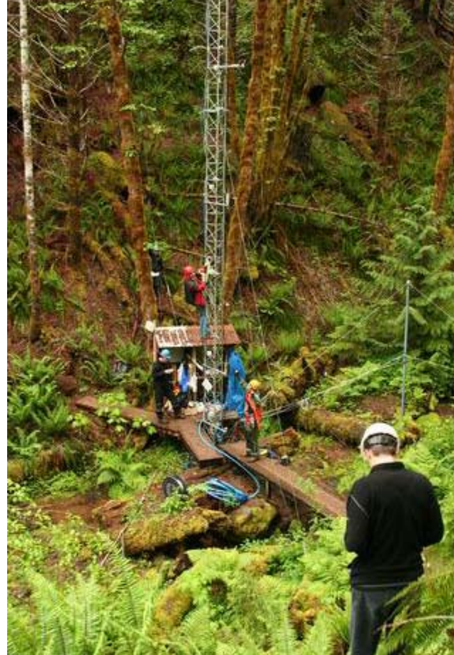
An international group of engineers, scientists and cable experts teams up in the H.J. Andrews Experimental Forest in June, stringing cable along a stream and, using a potato canon from a 100-foot tower, threading it through the old-growth canopy. (Photo: Lina DiGregorio)
