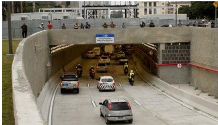
The tunnel "Via Expressa" in Rio
