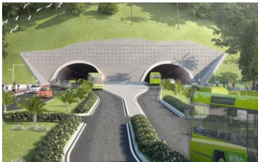
The tunnel "Charitas Cafuba" (under construction)
